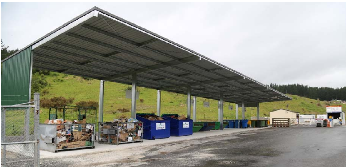
Figure 7 - Recycling Station at the Waitomo District landfill
