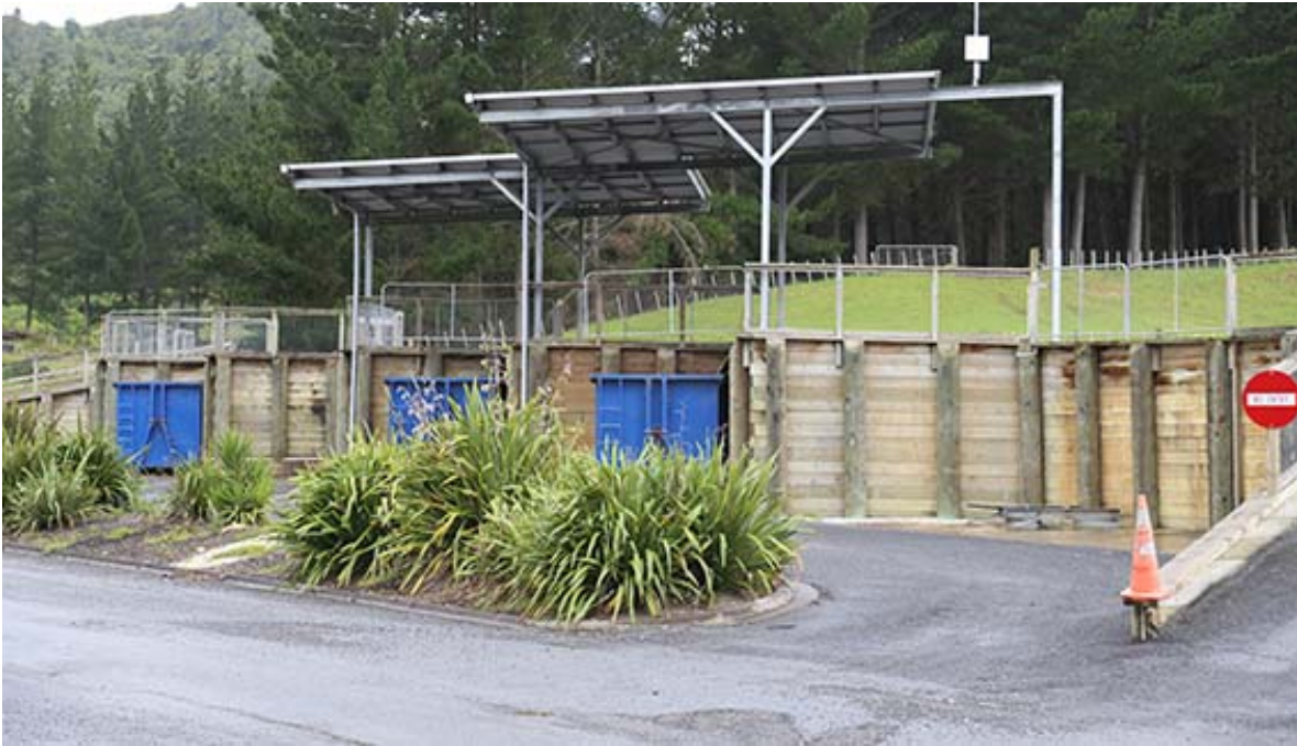
Figure 5 – Transfer station located at Waitomo District Landfill
